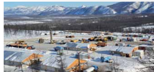
New community buildings at Ozerny, Khabarovsk Territory
