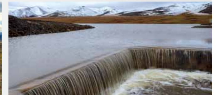
Tailing storage at Mayskoye
